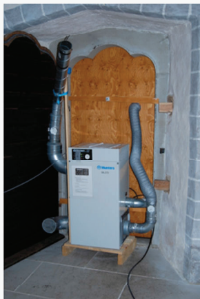
Sorption dehumidifier, temporary installation in a church on Gotland
