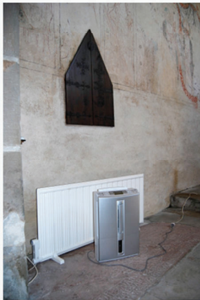
Condensing dehumidifier used during summer in a church on Gotland
